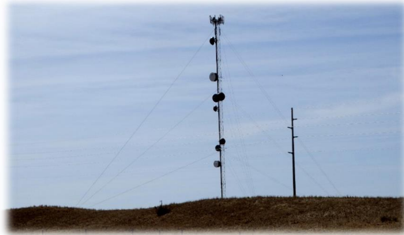
Cell tower-Highway 2-East of Dunning
